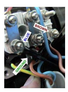
**Style 1 Motor and Wiring**
