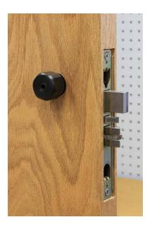
Thread the drill guide in until it makes contact with the inside of the mortise pocket.
