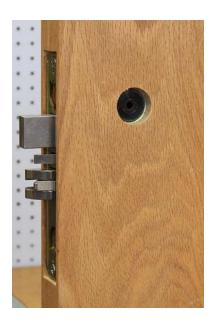
When the hole is drilled, remove the HIT-21 drill guide.
