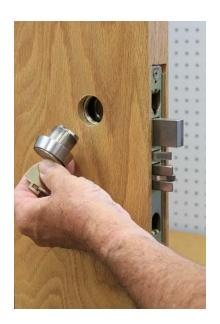
Next remove the outside mortise cylinder and replace with the HIT-21 drill guide.
